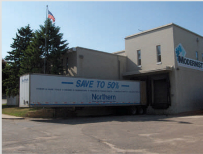
Rear Dock area of Building
