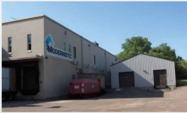
Side of Building with Storage Area
