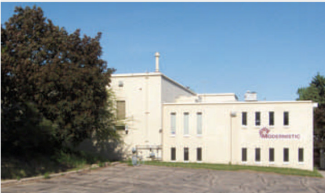
Front of Building
